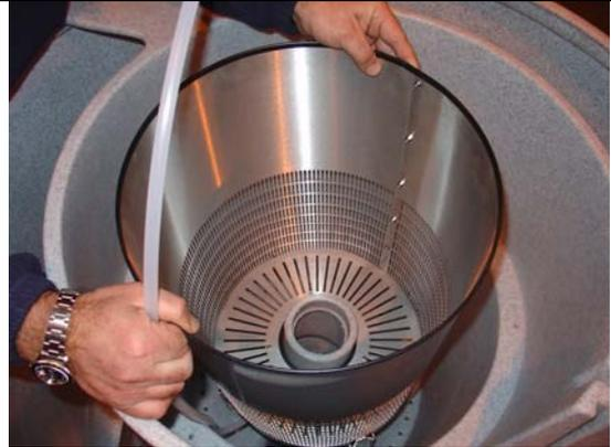
10) Align the air tube as shown, ensuring that the "Eazy" support legs are positioned equally either side of the waste drain.
